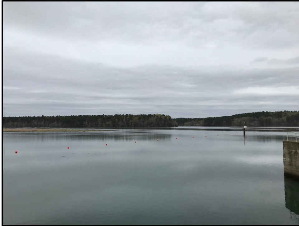
PHOTO 4-4 UPSTREAM OF DAM
