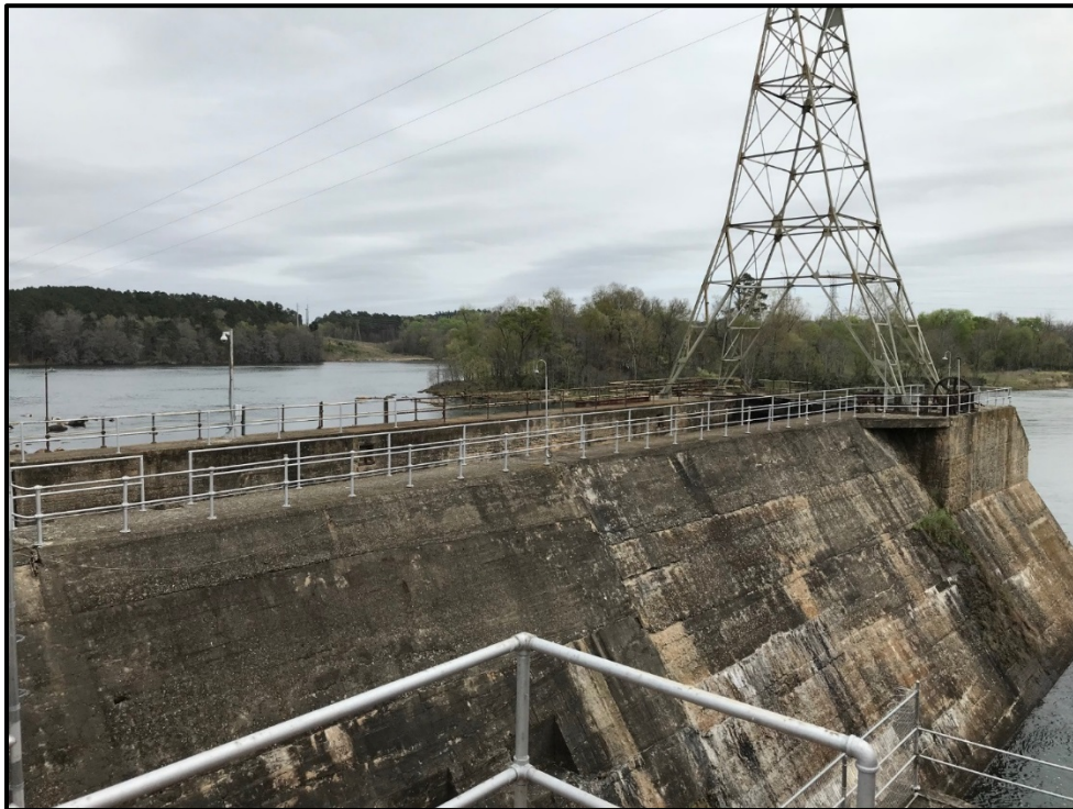
PHOTO 4-3 NAVIGATION LOCK, VIEW LOOKING DOWNSTREAM
