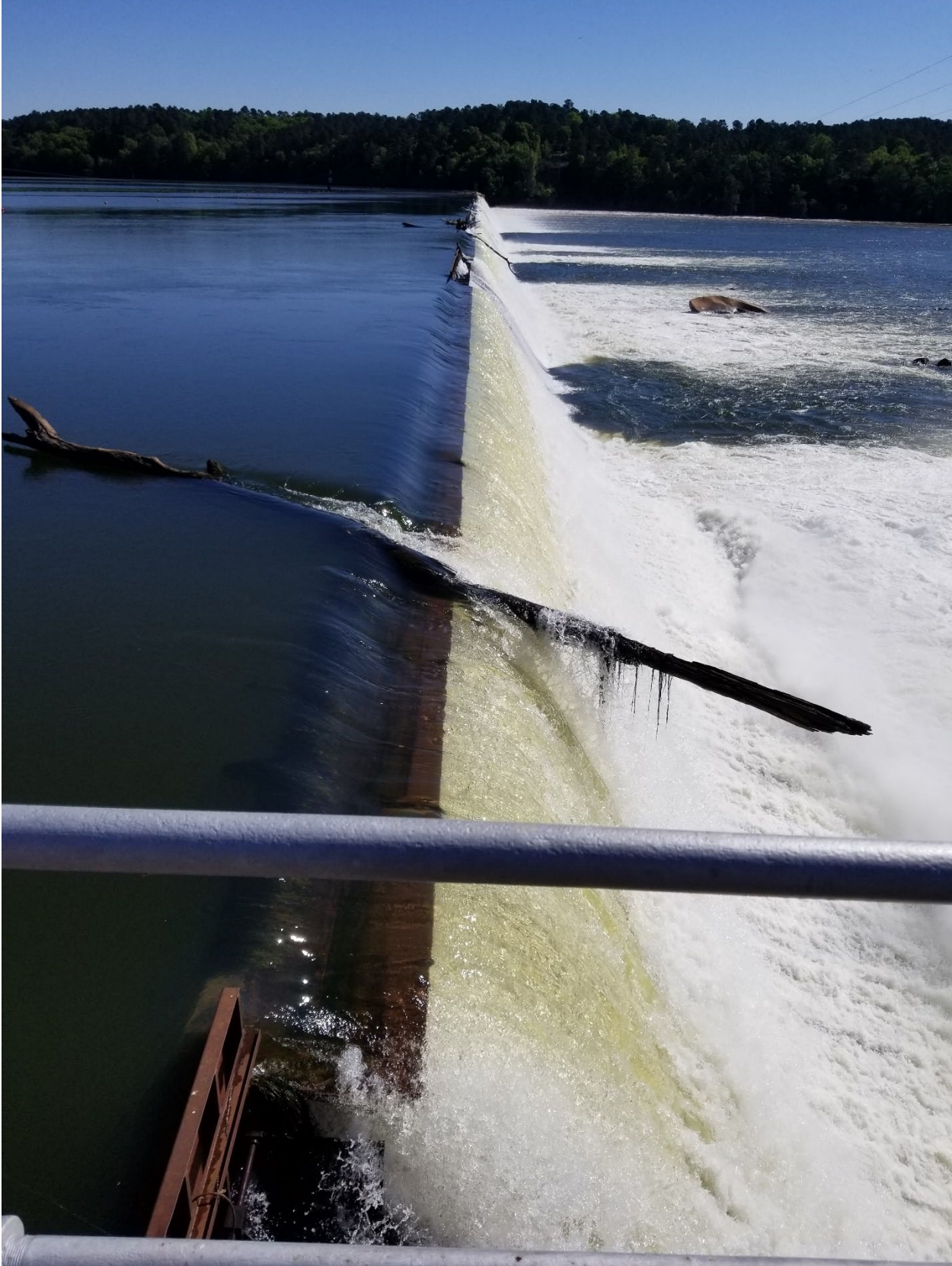
FIGURE 4.17 STEVENS CREEK DAM, VIEW LOOKING FROM GEORGIA TOWARDS SOUTH CAROLINA
