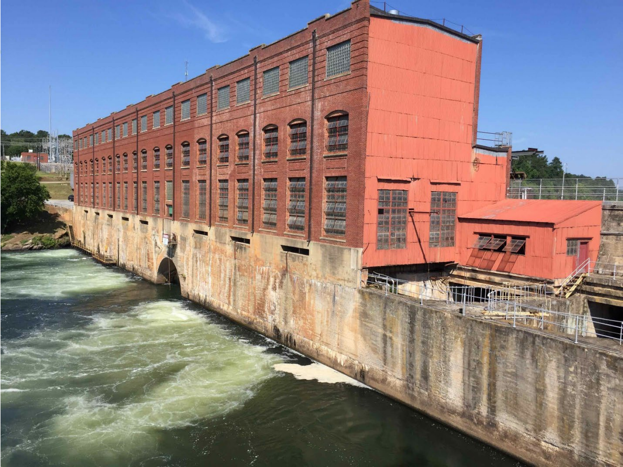
FIGURE 4.16 STEVENS CREEK PROJECT POWERHOUSE
