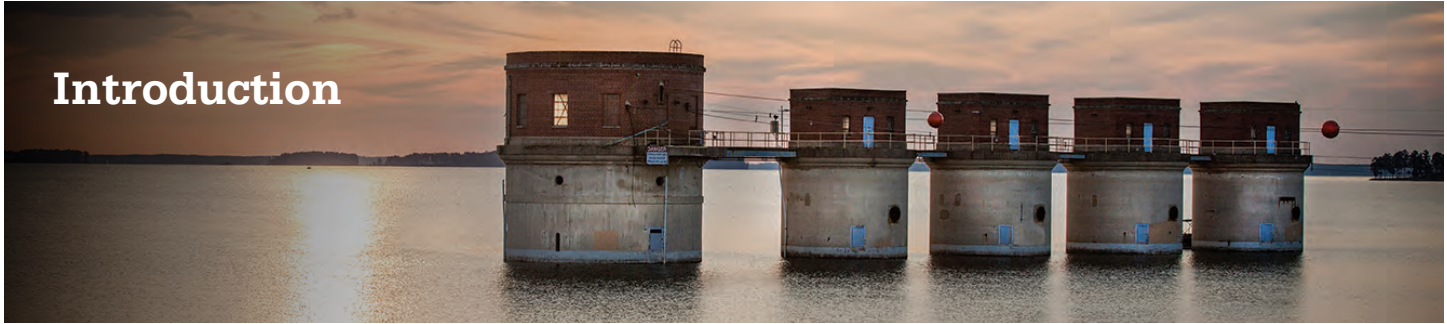
Intake towers at Lake Murray, SC
