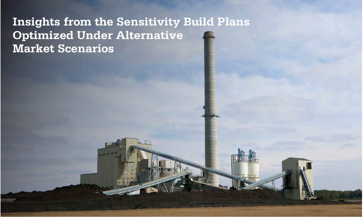
Cope Station; Cope, South Carolina
