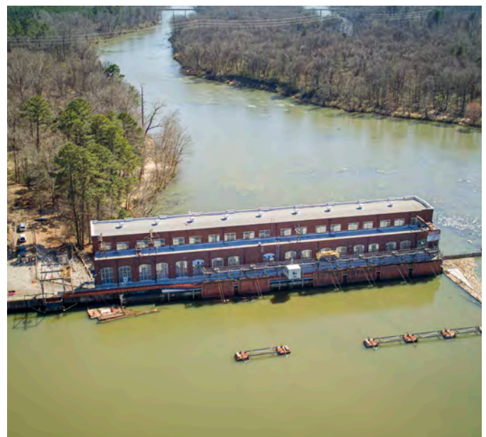
Parr Hydro Station; Fairfield County, SC
